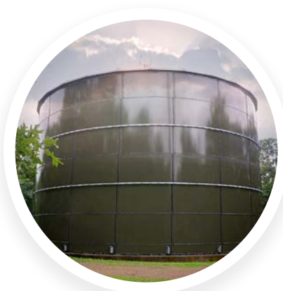
Ground Storage Tank
